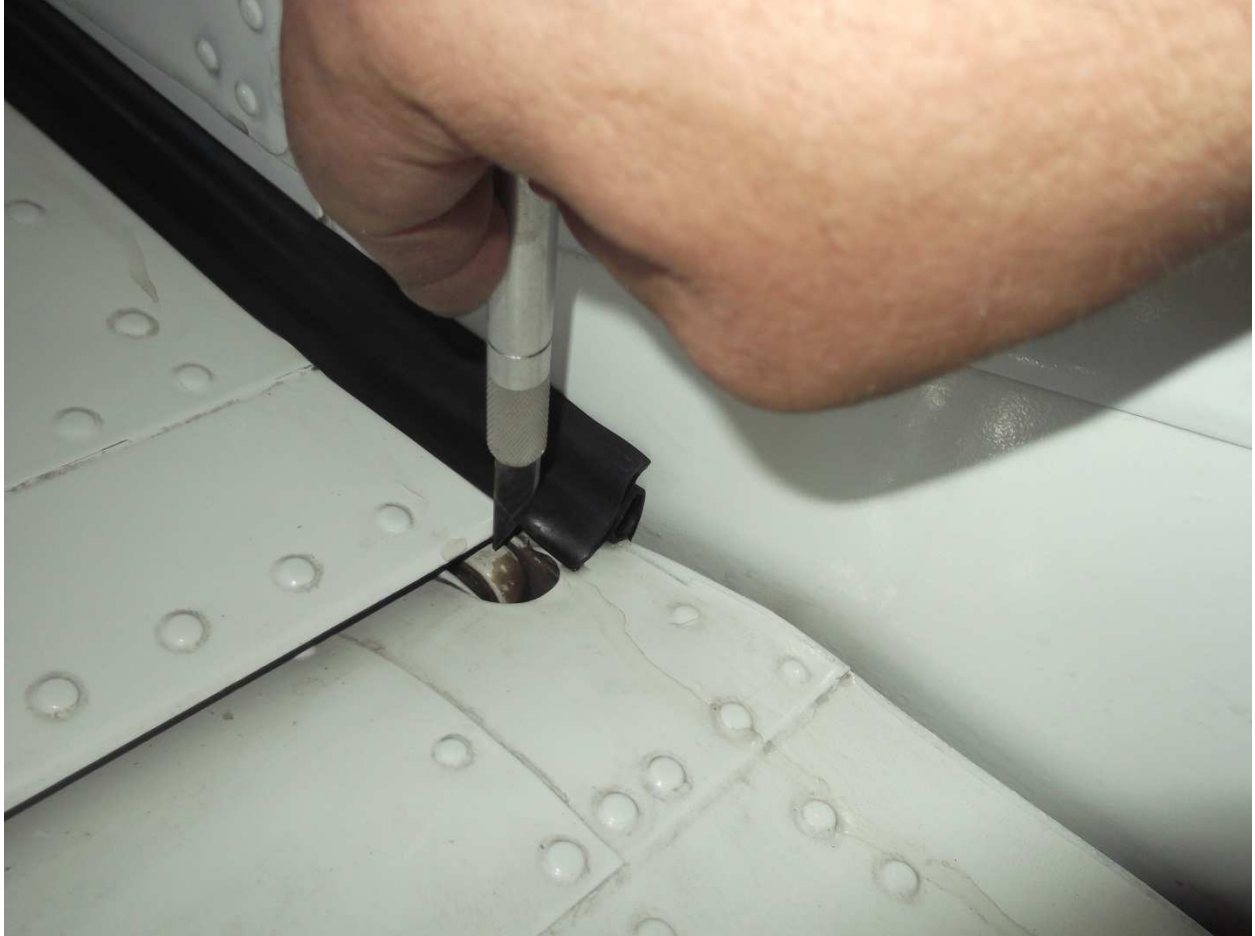
I left the new seals long until they were completely installed, then trimmed the excess (top and bottom).
