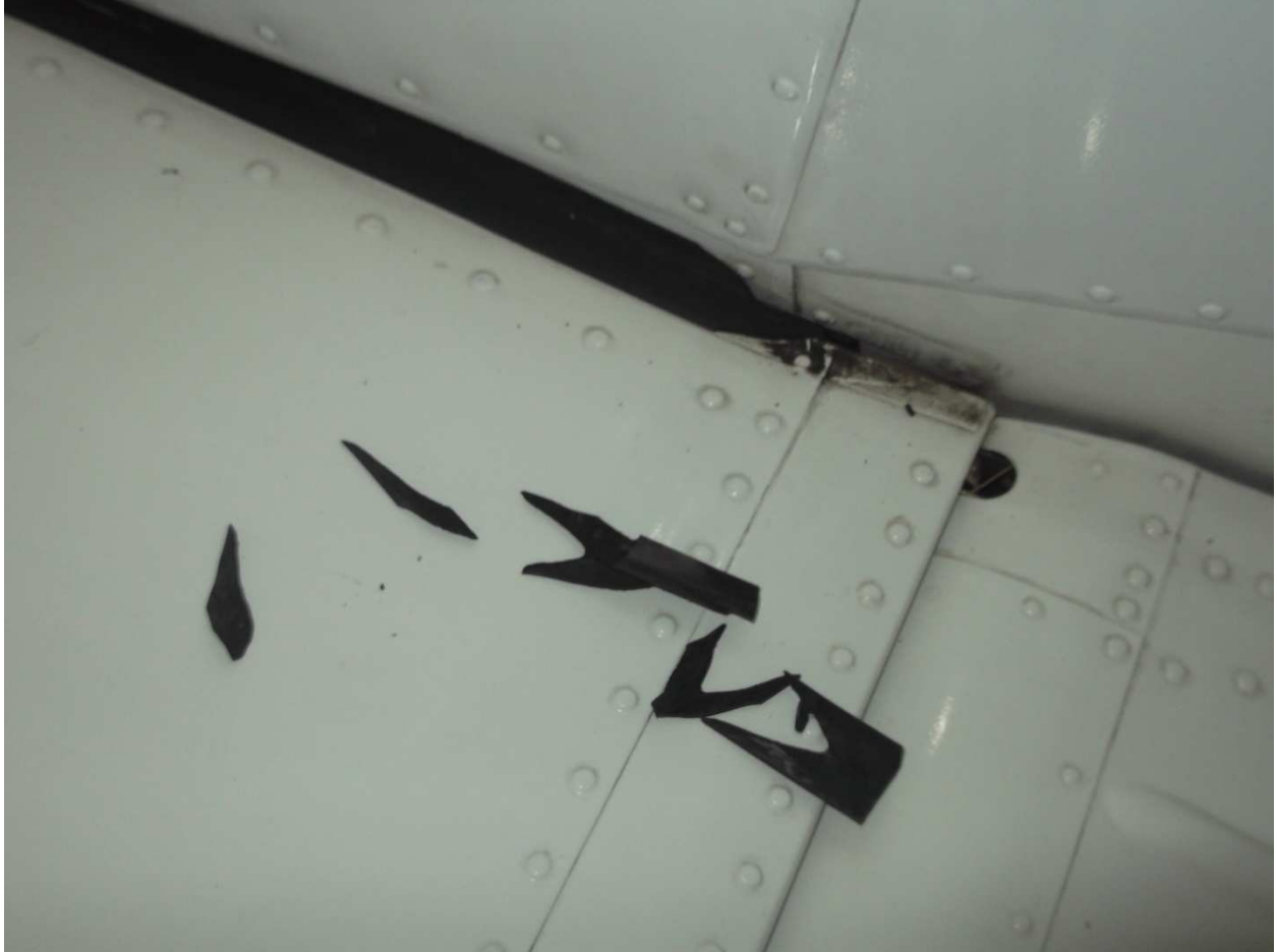
Removal of the old, crumbly wing root seal took more effort than expected.
