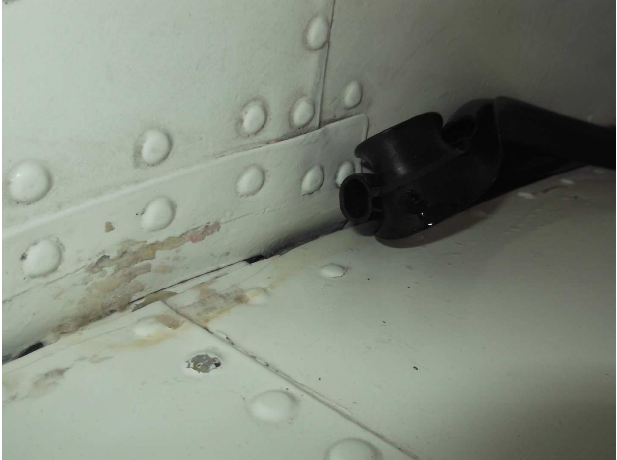
I trimmed the bulbs from the seals where they passed over or under the wing spar.
